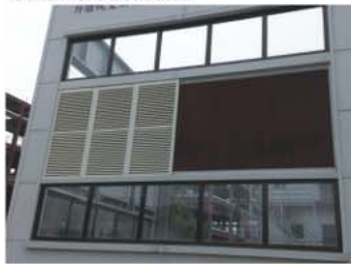
Whole plant with cooling pads and air intake shutter.
