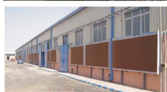
Whole plant with cooling pads and air intake shutter.
