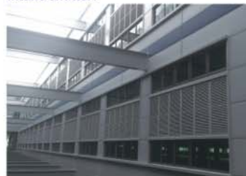
Whole plant with cooling pads and air intake shutter.
